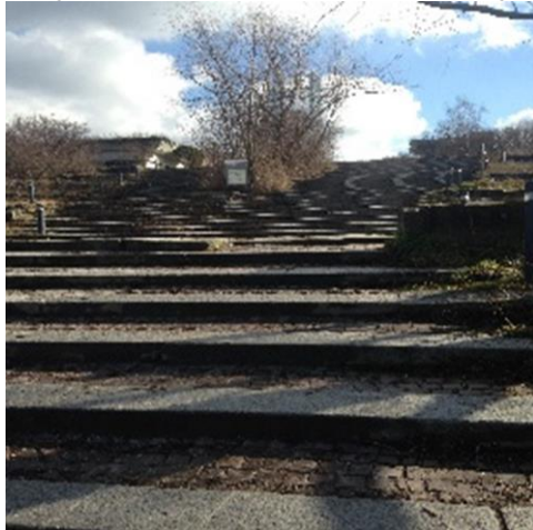
Figure 4: The area for outdoor stairs walking
